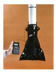
4.9 When the hub is heated to the correct temperature, unplug the heater. Remove the insulation/bag, special heater coil and the thermocouple.
