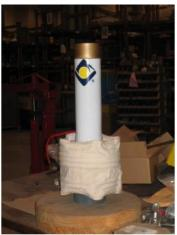
3.7 Cover hub with insulation or supplied bag in tool kit.
