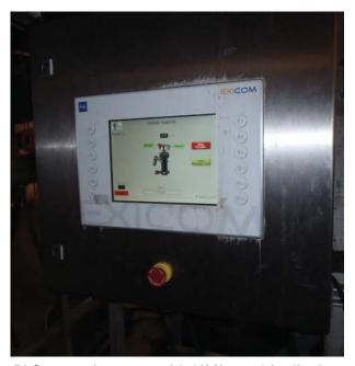
PLC control system with HMI graphic displays.
