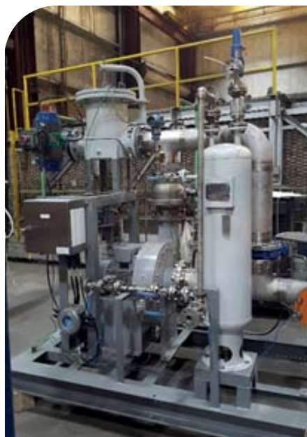
Induction fan module for fugitive dust extraction and capture
